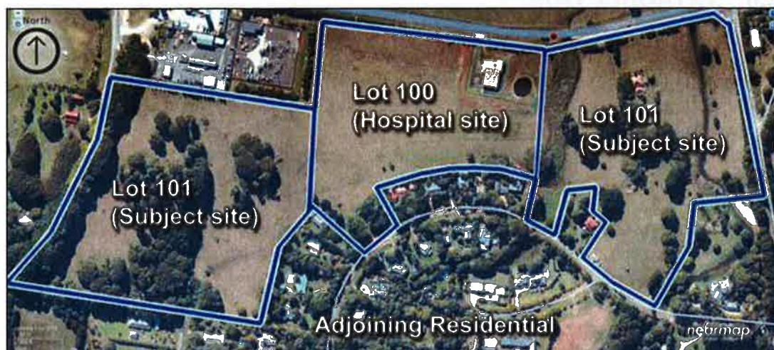
Figure 2 – Aerial Site Overview (Source: Nearmap.com.au image dated 3 July 2012; sourced 30 October 2012)
